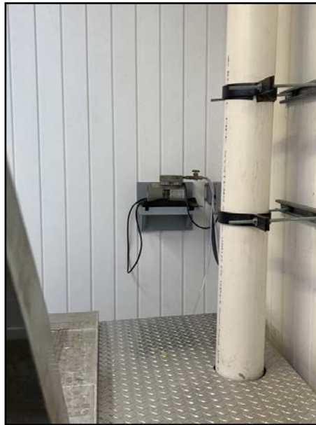
To oxygenate the water, a small compressor pumps air through a hose lying along the bottom of each tank.
